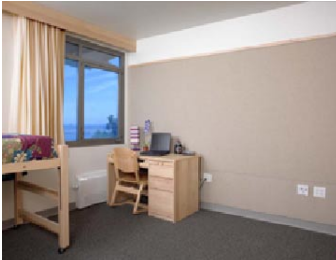
Student Housing - 1/2" tackable/acoustical - 5 1/2' and a 1 1/2' horizontally rail roaded band
