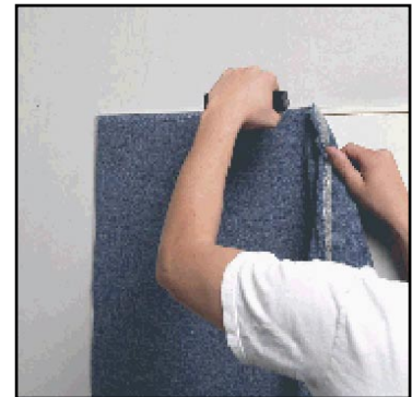
Step 3; fabric is secured into the track's locking jaws. The FABRICMATE System holds the covering firmly in place, while allowing it to be easily removed and replaced if needed. (100% recycled - Terratex® covering shown)
