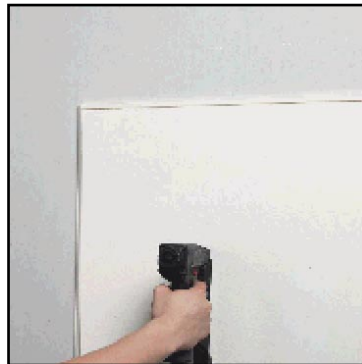
Step 2; core material is placed inside the tracked area. (1/2" Flametack shown)
