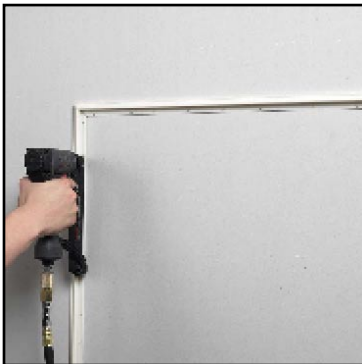
Step 1; "Track" is laid around the perimeter of the area to be covered. (1/2" Beveled Track shown)
