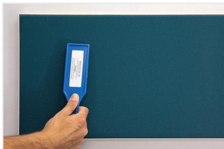
Once the Fabric is all rolled in, you can make minor adjustments by using the Fabric Stretcher Tool. **Use sparingly as is only meant for minor adjustments. If used excessively or incorrectly it can damage your Fabric.**
