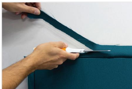
Once the Fabric is fully tucked in (including corners) and the panel/area looks good, trim the excess Fabric from around the panel/area edges leaving about 1/4" to 3/4" hanging out.
