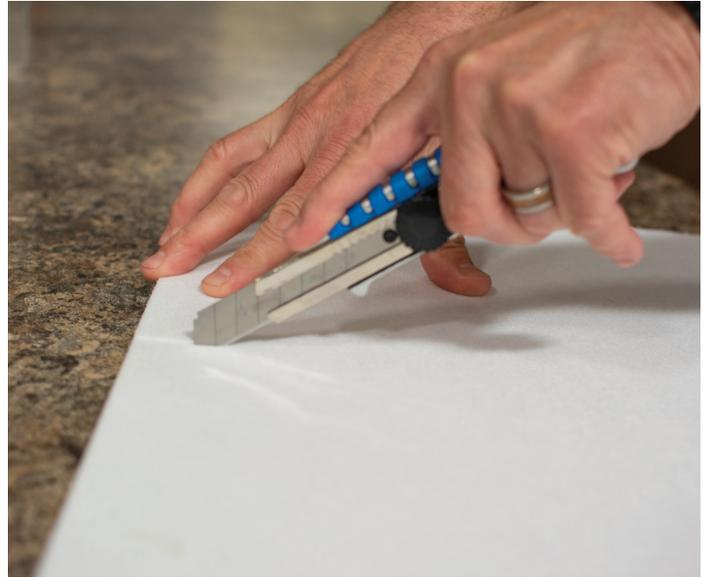
Use a Utility Knife to cut the Backing to size so it sits in the Frame flush and can be covered by the Fabric.
