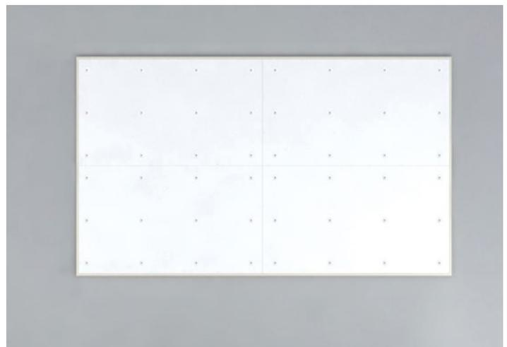
Use 7/8" 1/4" Crown staples roughly 12" apart to fasten the Backing to the wall.
