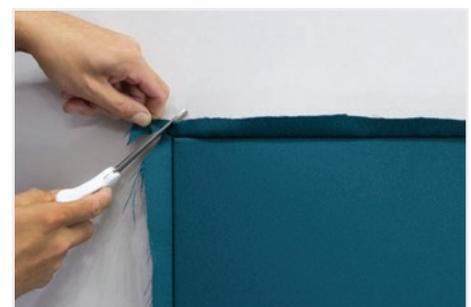
Trim the excess Fabric on the corners of the panel/area by cutting within a 1/4" of the corner.
