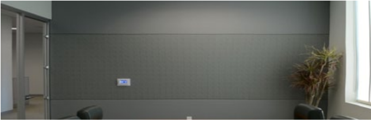
Conference room with three 1/2" thick tackable/acoustical railroaded bands with Anchorage Slate and Rock Star Frost fabric
