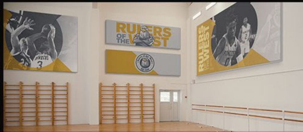
Custom Printed Site-Fabricated Panels in Gym
