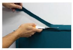
Once the Fabric is fully tucked in (including corners) and the panel/area looks good, trim the excess Fabric from around the panel/area edges leaving about 1/4" to 3/4" hanging out.
