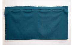
Start by ensuring your Fabric will cover the panel or area you are installing on with 2" - 4" extra over each side. Use the Rocker Tool to lightly press Fabric into jaws assuring it's straight and even across the top.
