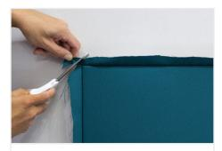
Trim the excess Fabric on the corners of the panel/area by cutting within a 1/4" of the corner.
