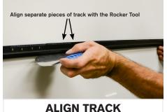
Fit the Rocker Tool into the Frame jaws to align and hold each new piece of Frame to the previously mounted piece. SNAP LINES
