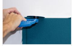
Use Corner or Rocker Tool to tuck in corners first. Then use Roller Tool to roll the remainder of Fabric into the frame jaws, hiding the excess. Very gently lean Roller Tool to the sides of the jaws while rolling for better results.
