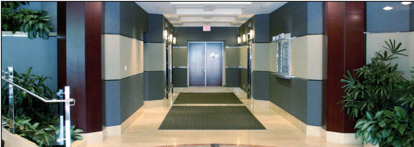
Acoustics and Wall Protection in Lobby / Hallway
